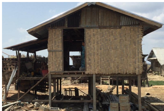
New IDP shelters being constructed in Rakhine. May 2015. Credit: OCHA
