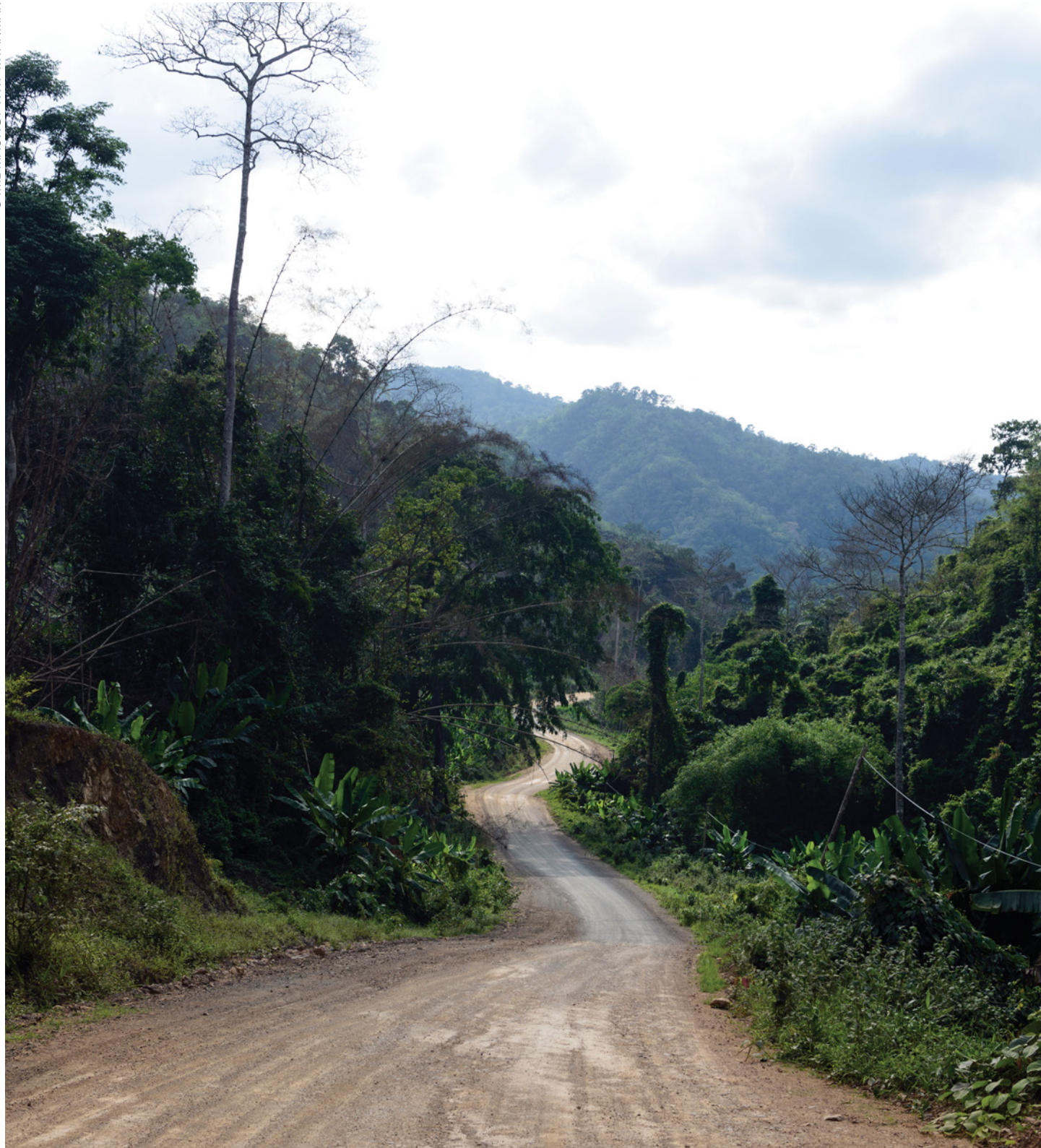
The current access road for the planned Dawei road between the Myanmar-Thai border and the village of Myitta.
