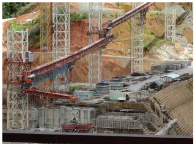
Photo: Paunglaung dam under construction (pre-2015).
