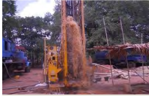
Photo 54: Irrawaddy Fm. Aquifer Development, Myaynegyi Village. Source: DRD
