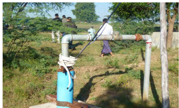
Photo 59: Thazi TWS, Northeast Wellfield, Nov. 2016
