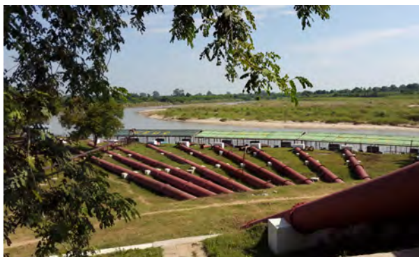
Photo 6: Irrigation Pumping Station on Mu River, Ayadaw
