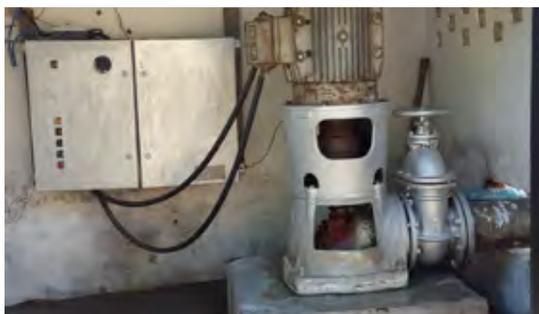
Photo 44: Electro-Turbine Pump, Monywa Irrigation Area
