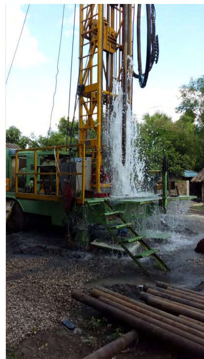
Photo 42: Airlift Production Tubewell – Twin Taw Village, 2016
