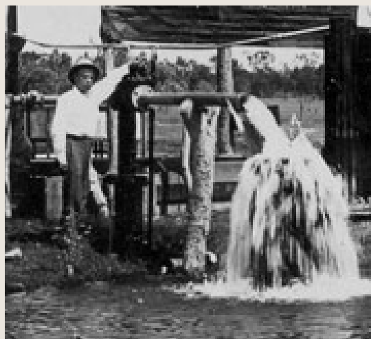
Artesian bore Balcaldin, Queensland (detail) c 1907, Mobsby Coll, Fryer Lib, Brisbane. Source: www.rlms.com.au
