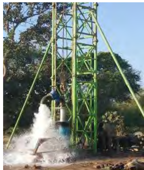
Photo 68: Developing Deep All. Aquifer, Mandalay. Source: MDC
