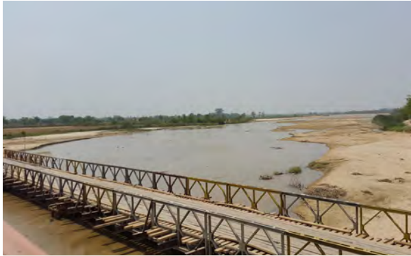
Photo 24: Exit of Yin Chaung from Sub-basin – Dry Season 2017
