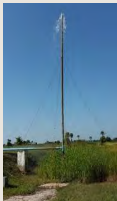
Photo 50: Myay Net No. 1 Irrigation DTW. Pressure Head > 50 m
