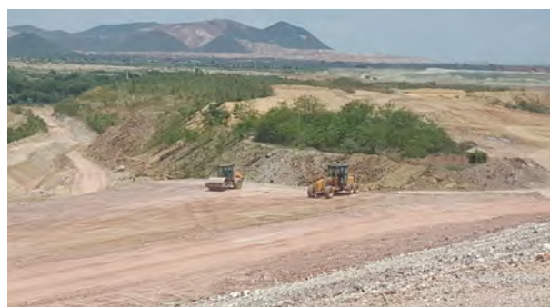
Photo 13: Letpadaung Taung Copper Project.
