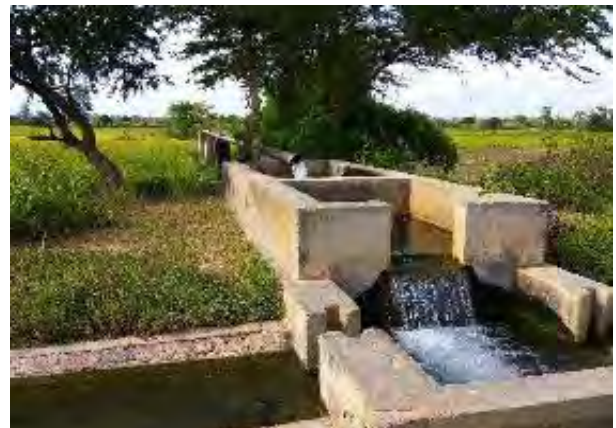
Photo 39: Ywahtaung Irrigation DTW, Y/A Aquifer Yinmabin
