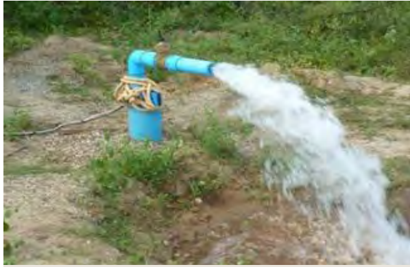
Photo 53: Sharkey Irrigation Tubewell, Palin Village
