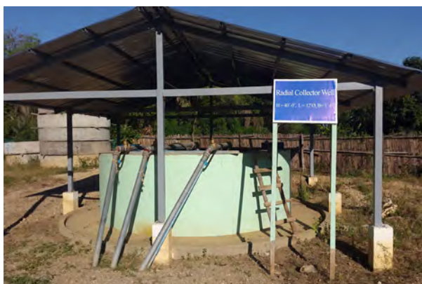
Photo 22: Minbu Town Water Supply Collector Well System
