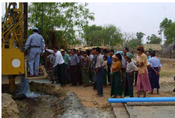
Photo 16: Drilling of New Tubewell. Source: U Ngwe
