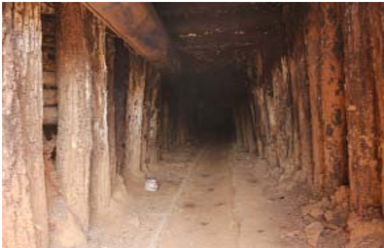
Logs are used to prop up the roof in one of the Mawchi mine tunnels
