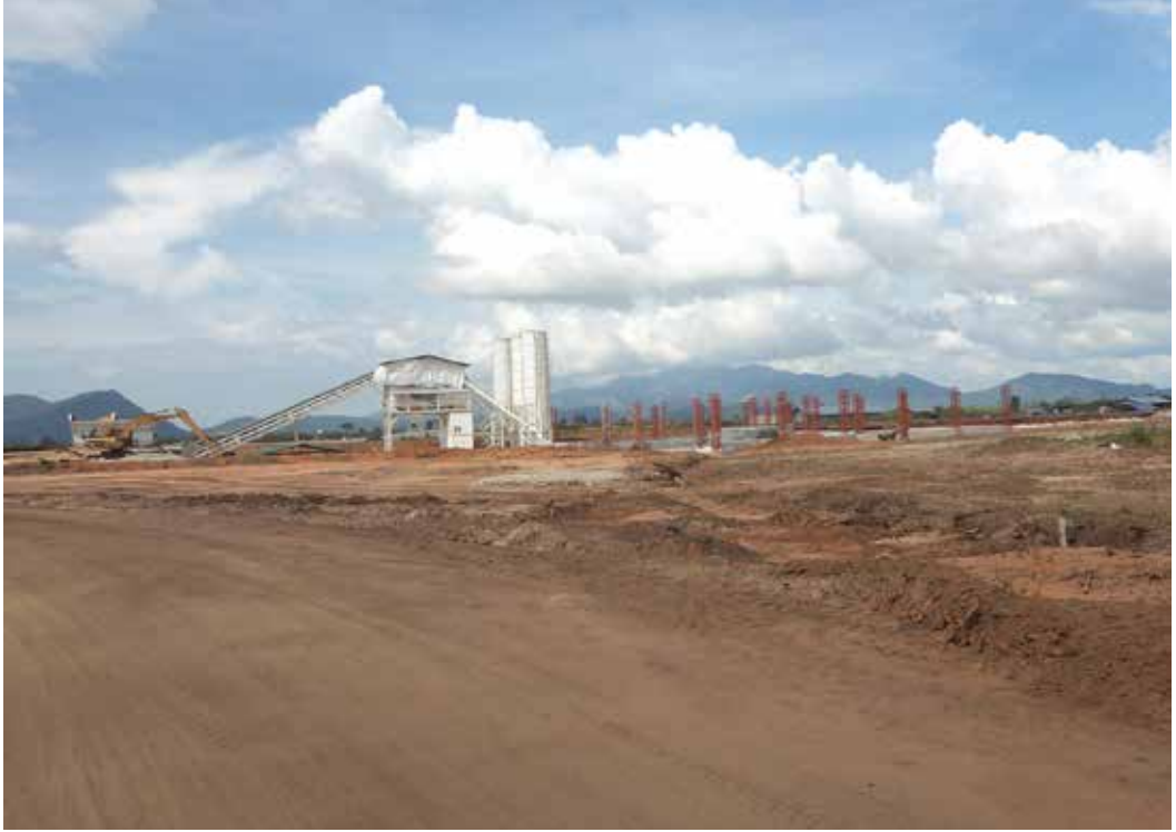
Project construction near Ngapidat village
