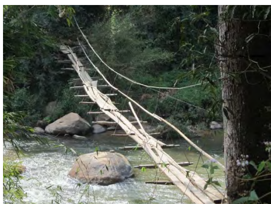
Local bridge in East Shan, Myanmar, 2015
