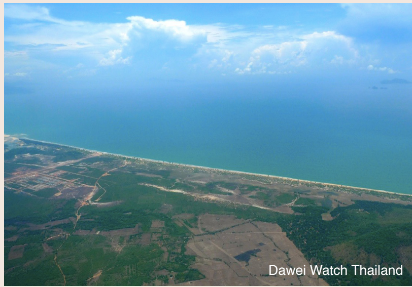
The Dawei Deep Seaport and Industrial Estate Development Project site.
