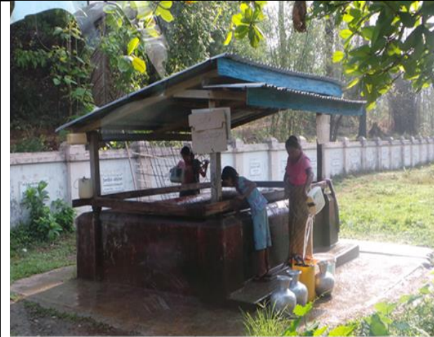
Protected Dug Well
