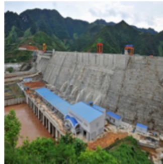
Hydropower and energy
