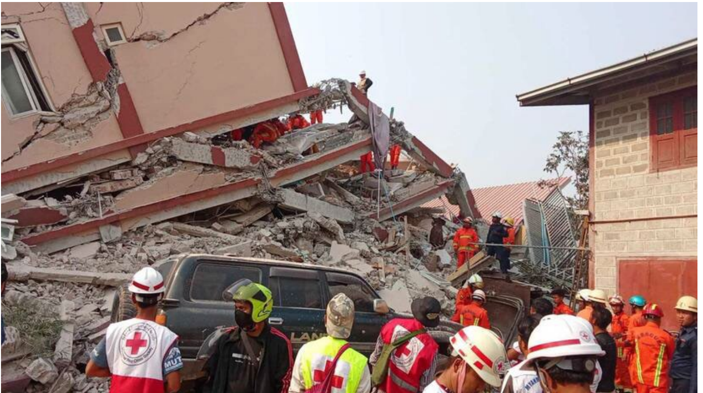
Rescue teams from the Myanmar Red Cross Society look for survivors in a collapsed building following a 7.7 magnitude earthquake in central Myanmar on 28 March 2025. (Photo: Myanmar Red Cross Society)
