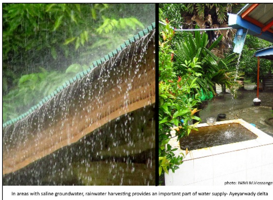
Figure 3.10.4-b – Ayeyarwady Delta, in Kyaiklat town (loc.: 16.444, 95.725): Due to high salinity in groundwater and surface water, some communities rely nearly exclusively on rainwater harvesting.
