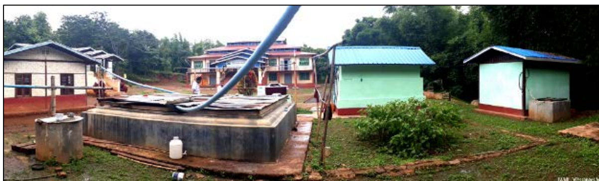
Figure 3.7.5-b – Plateau Limestone: Large-scale rainwater harvesting was installed in 2007. Then in 2016 a 250 m tubewell was drilled by IWUMD, with a yield of 4.5 m 3 /h. Loc: 20.876°, 96.766° (photo: Viossanges)
