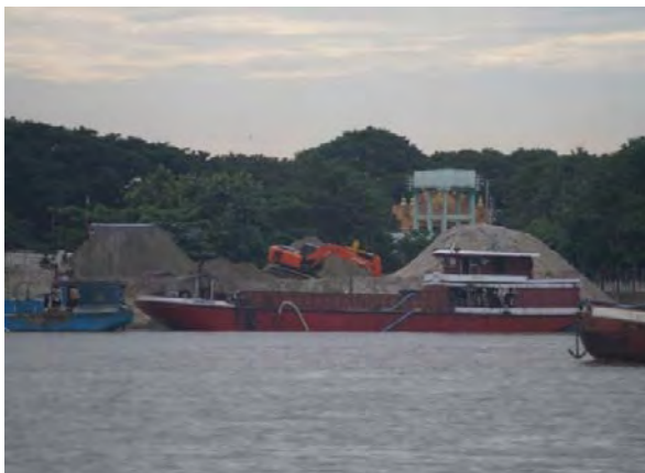
Figure 147 - Sand being moved by an excavator, near Mandalay
