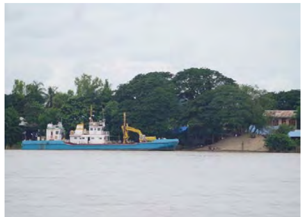
Figure 148 - Example of excavator aboard a vessel
