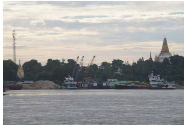
Figure 146 - Floating cranes on barges at Sagaing
