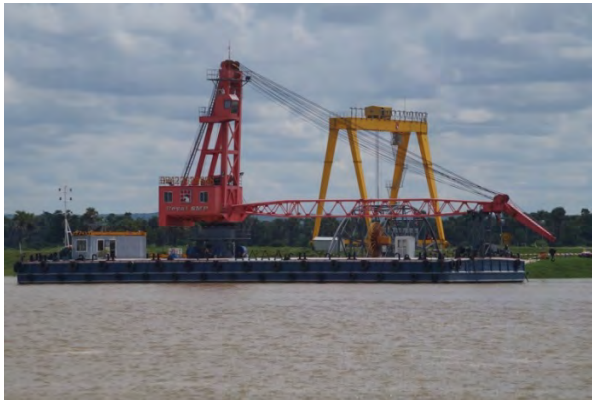
Figure 145 - Gantry crane and barge crane at Semeikhon
