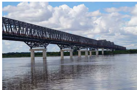
Figure 144 - Ayeyarwady River Bridge at Pakokku (Study Team)
