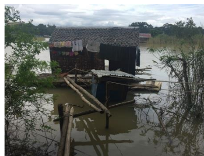
Figure 21 - House located in an erosive river bend
