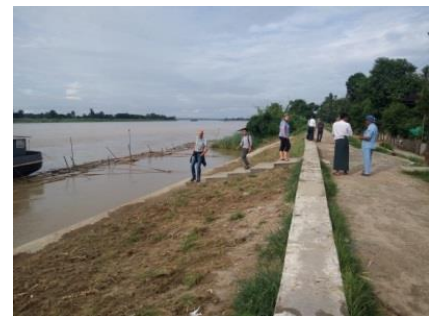
Figure 53 - Embankment at Nyaungdone
